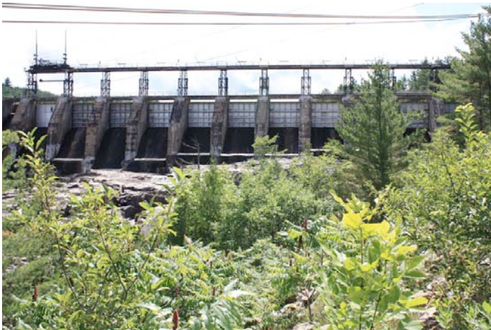
Barrage High Falls, Bowman.
